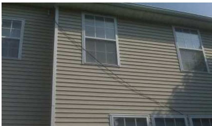
Fig. 3 Back of house to attic
