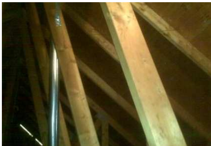
Fig. 4 Attic shot, some metal and one wire leg
