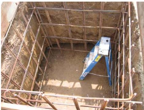
*A big hole in the ground for a 64' tower. Note the bell shape flare at the bottom.*
