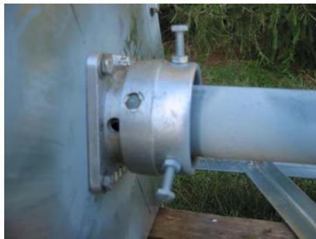
*Second thrust bearing detail. Note the hole drilled through the side near the base for a pin in case the rotor has to be removed for service.*
