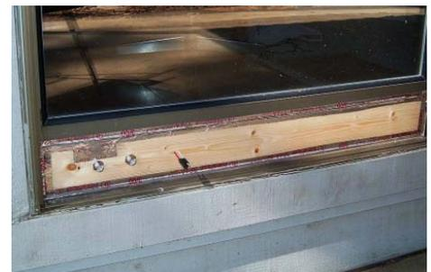
Since the window is partially open, you now have a gap between the glass in the lower sash and the frame of the upper sash (or the fixed frame of a single-hung window). Use the foam insulation to plug this gap, making sure you also plug any side gaps between the sash and the frame track. The actual strip of installed insulation is partly visible along the upper edge
