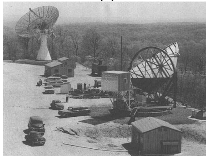
Figure 10. The Bell Telephone Laboratories satellite communications center at Crawford Hill in Holmdel, New Jersey, circa 1960. The steerable horn antenna used for receiving is to the right, while the sixty-foot (twenty-four) transmitting dish is in the upper left corner. (Courtesy of NASA, photo no. 227031)
